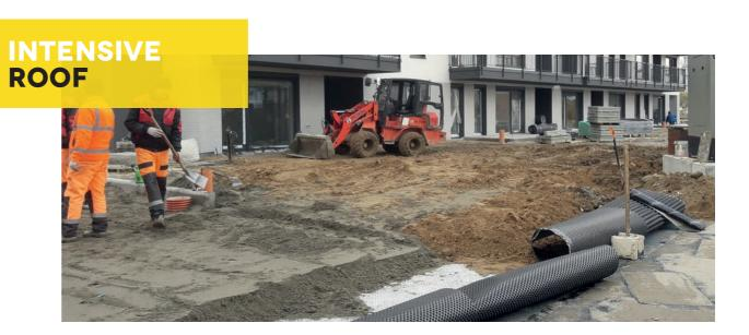
Heavy structure with functional purposes, usually placed on floor slabs of underground garages and terraces. It is implemented in order to restore the ground conditions in a given place, which will allow vegetation to grow. Intensive roofs also frequently include paths, playgrounds or recreational areas. The vegetation is made up of trees and shrubs, often in combination with ground covers. It is intended to resemble a garden or a square and therefore requires appropriate care and watering.
