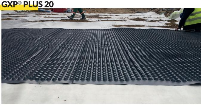
GXP® Plus 20 membrane made of high density polyethylene (HDPE), with a weight of 800-1200 g/m², is designed for mechanical and hydraulic protection of tunnels, green roofs or other underground structures with increased water flow.
