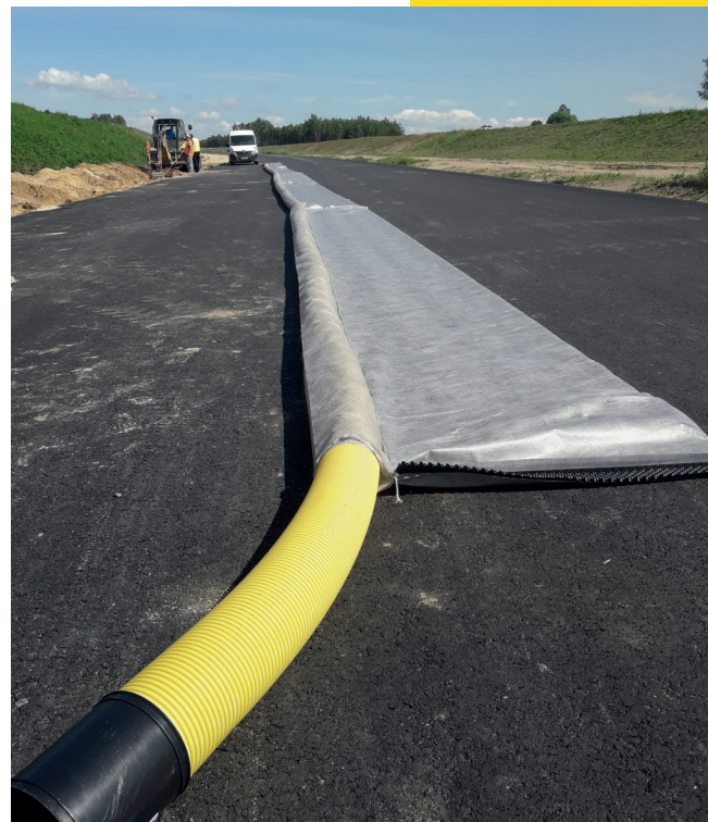
The mat is equipped with special geotextile sleeve in the lower part for the location and protection of the drainage pipe.
